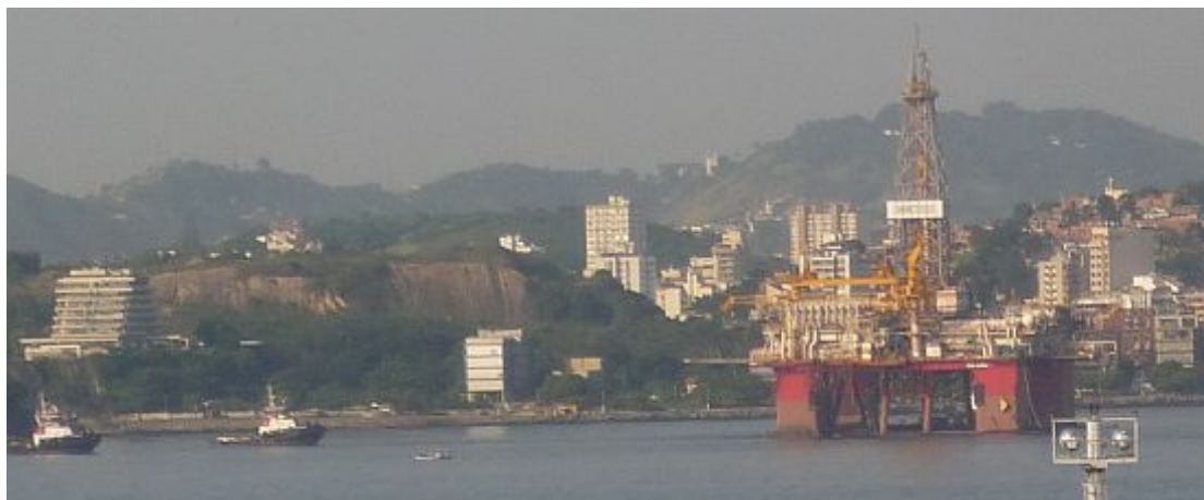
110614 Oil Rig Repair & Maintenance in Rio de Janeiro
