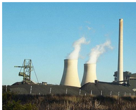
Bayswater Power Station.
