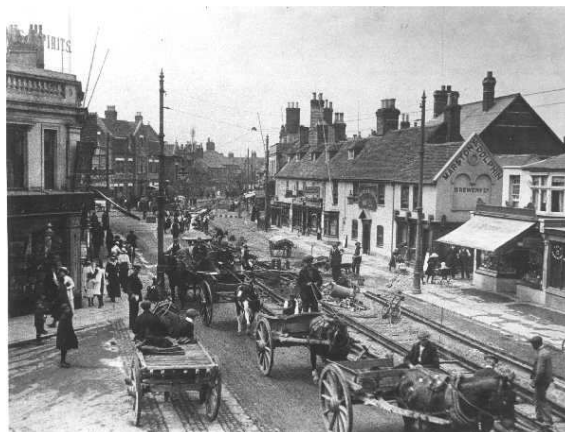
Laying the Tram Tracks near the end of the Horse-power Era
